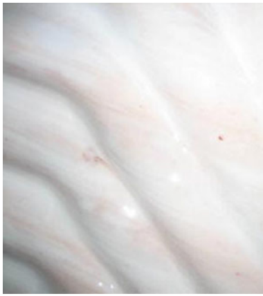
Fig. 5 Deposit attached on membrane water wall
